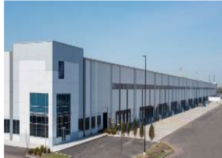
586 Gulf Avenue, Staten Island, NY
